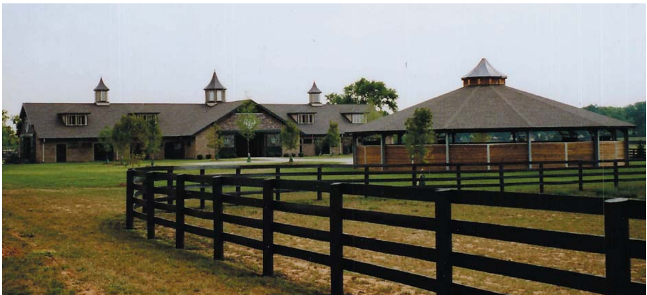
WINSTAR-Farm, Lexington, Kentucky, USA, Ceiling Mounted Walker with shingles
