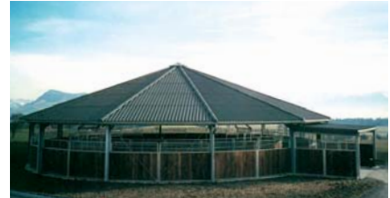
Paul Estermann Riding Sport Center, Hildisrieden, Switzerland, Ceiling Mounted Walker with corrugated cement fiber roof
